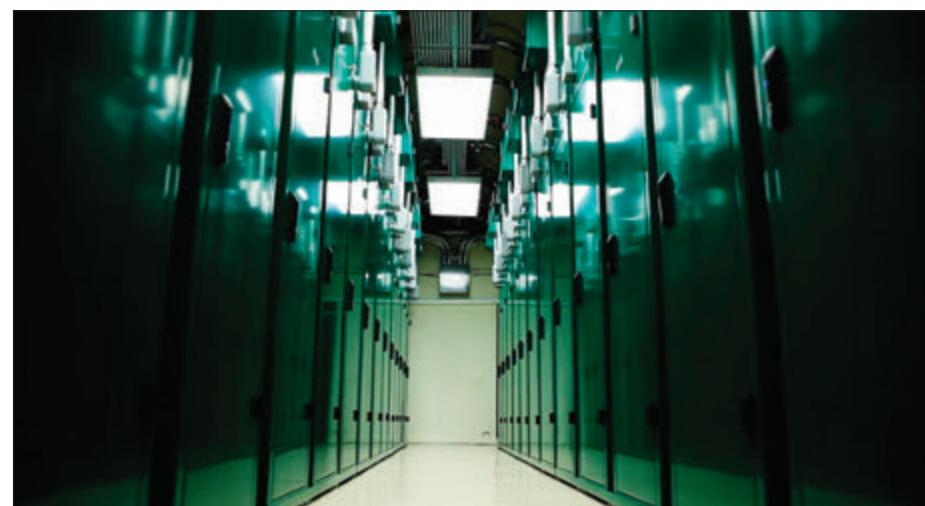
Our Green cabinets are self-contained and they hook into ceiling-mounted power, cooling and networking infrastructure that is enclosed in metal tubing. There are no exposed cables or wires, which reduces the risk of unauthorized tampering.
